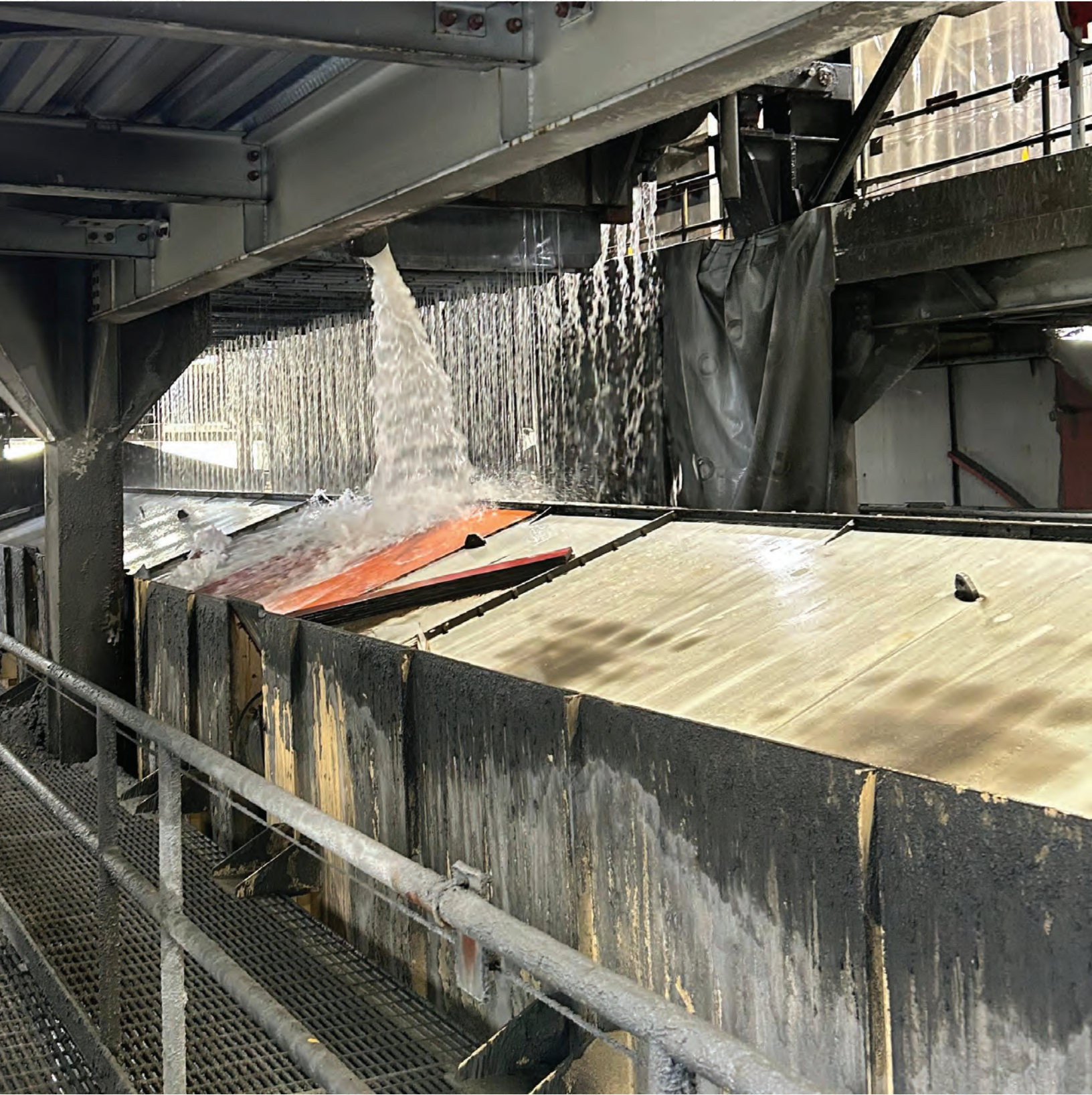
Water recovery at Cozamin dry stack tailings plant
