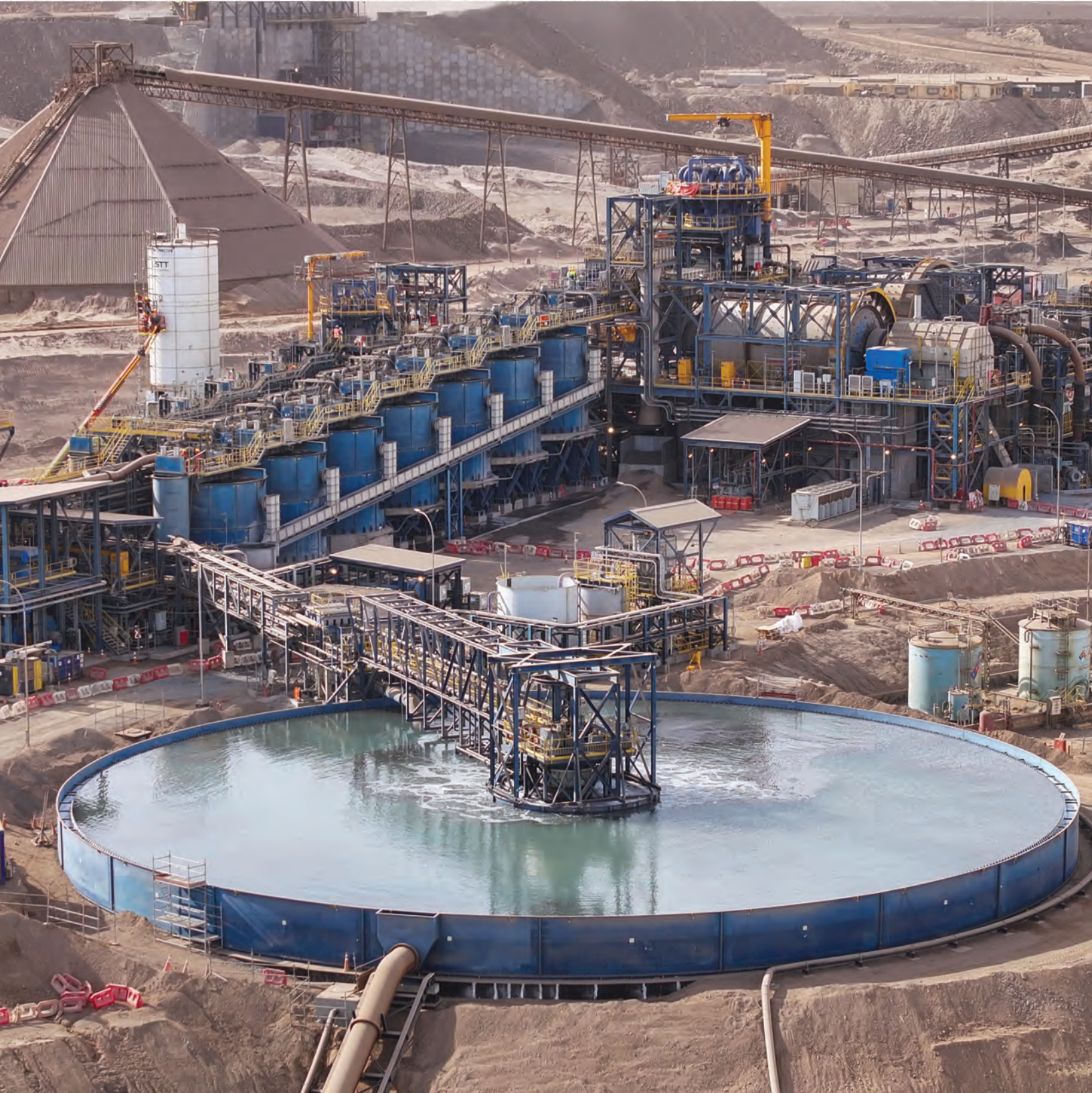
Tailings thickener, Mantoverde
