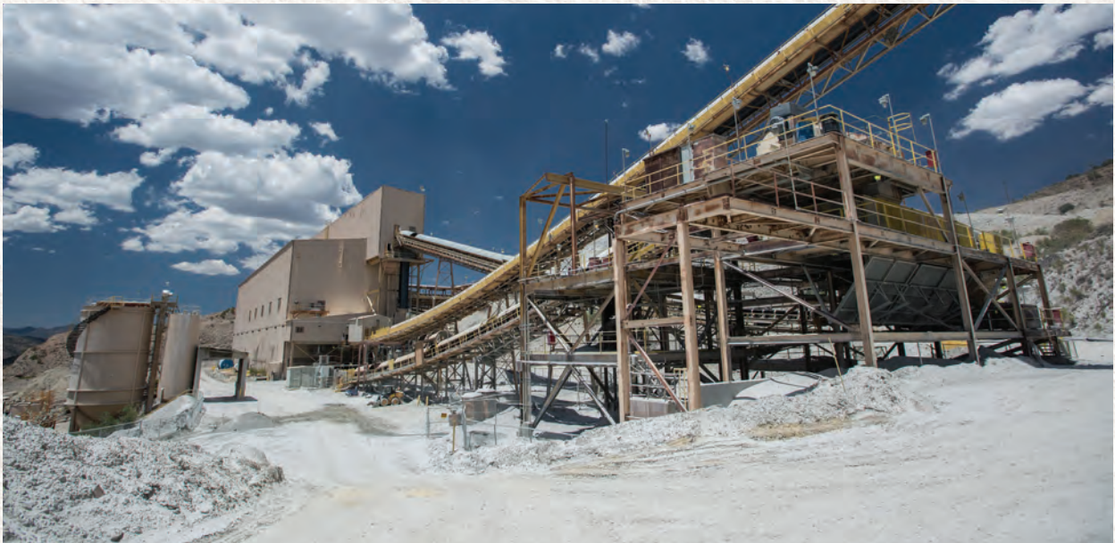
Secondary crushing circuit, Pinto Valley
