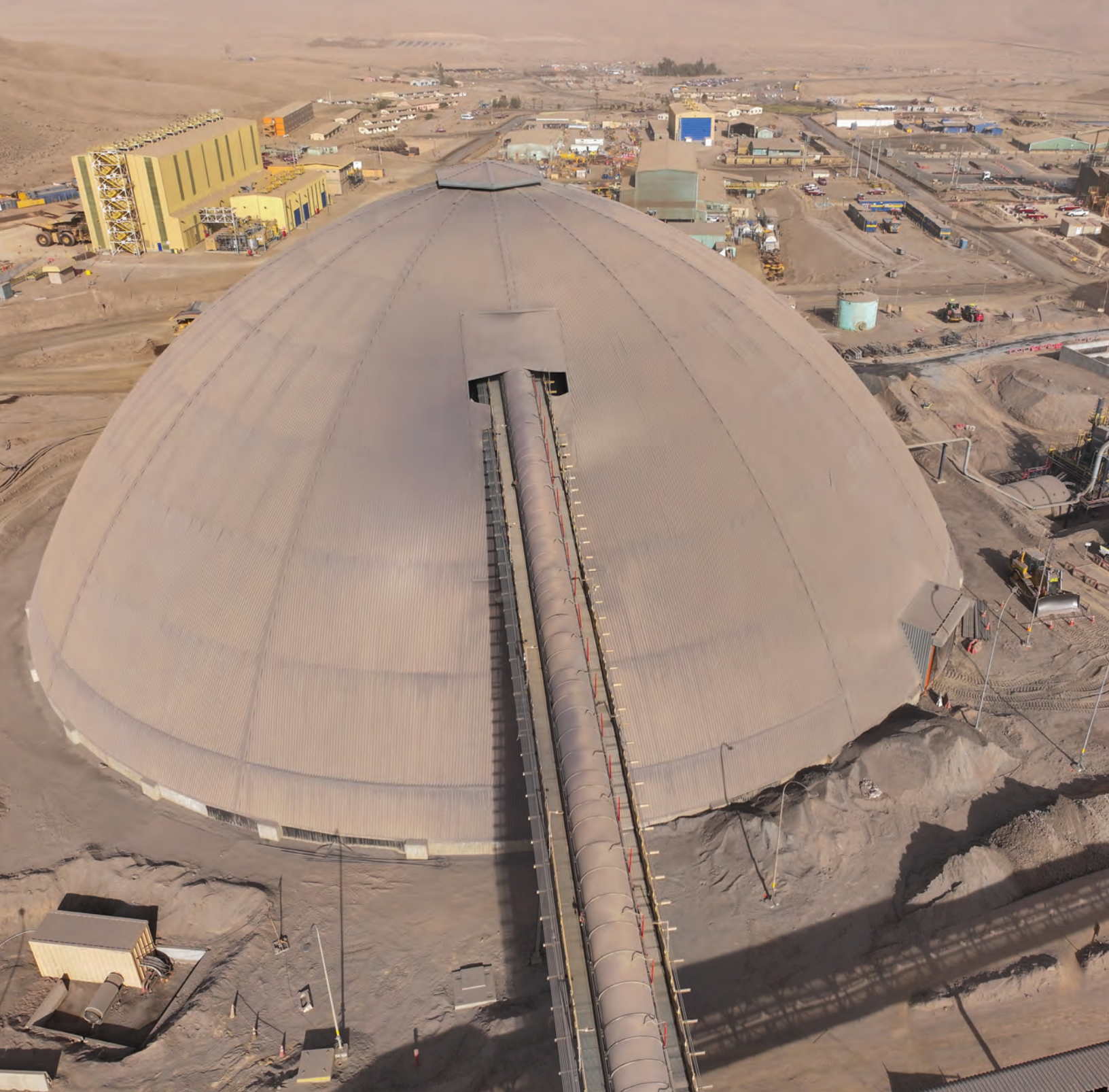
Covered coarse ore stockpile, Mantoverde
