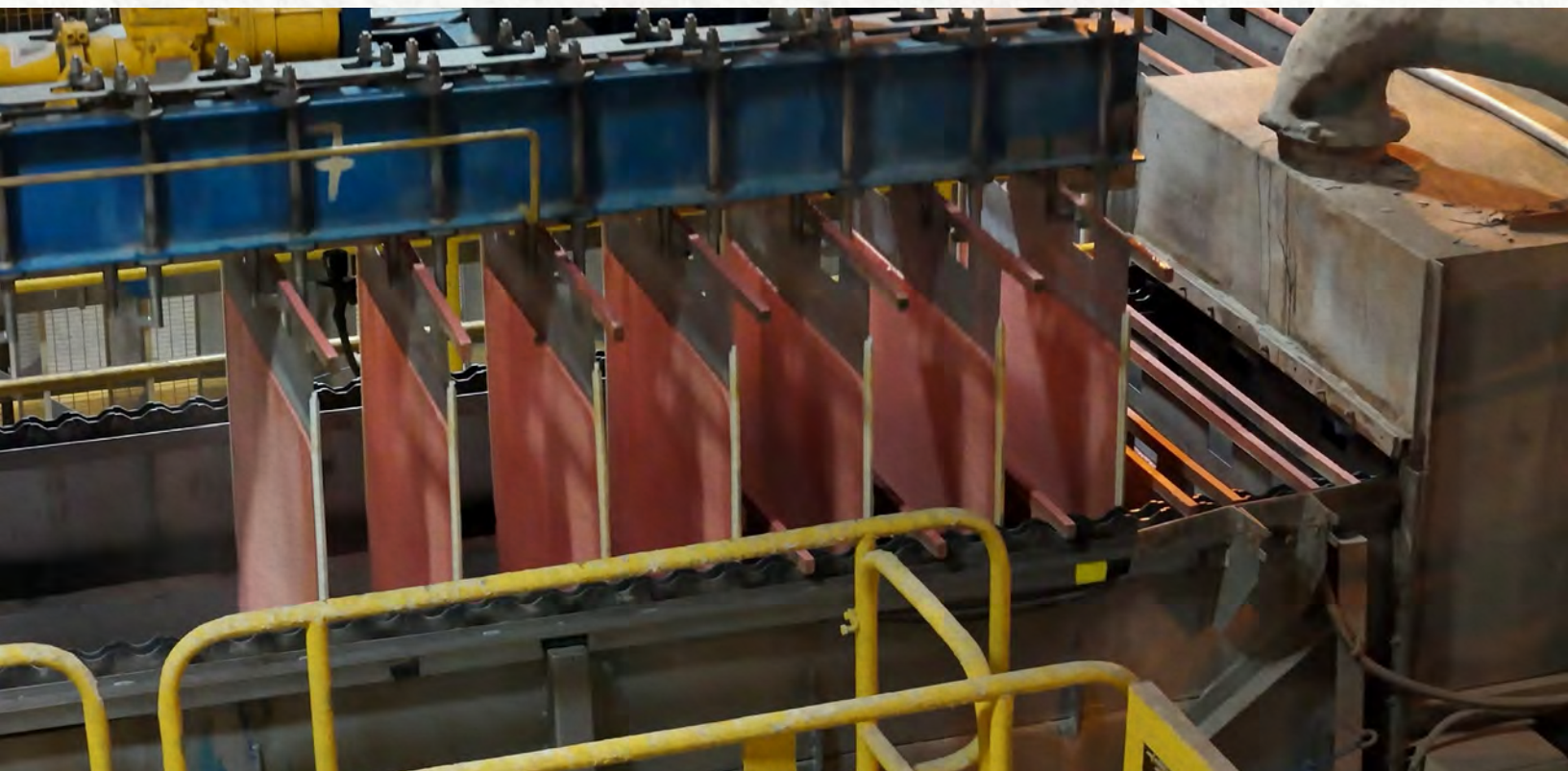
Mantos Blancos – Cathodes Collection at SX/EW Plant
