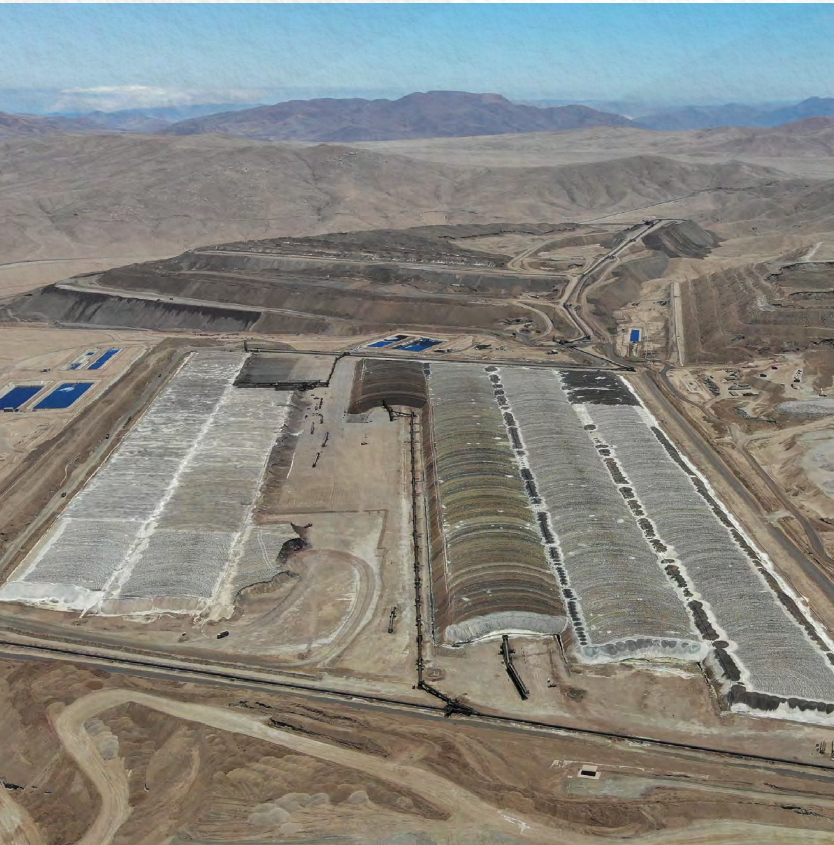
Mantoverde – Heap Leach Facility
