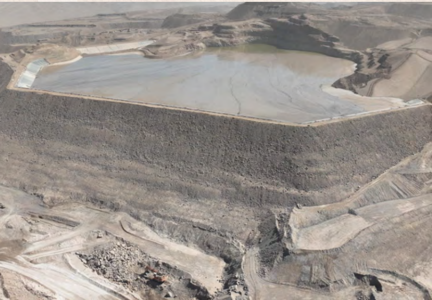
Mantos Blancos – Pit Phase 8, Stage 4 Construction
