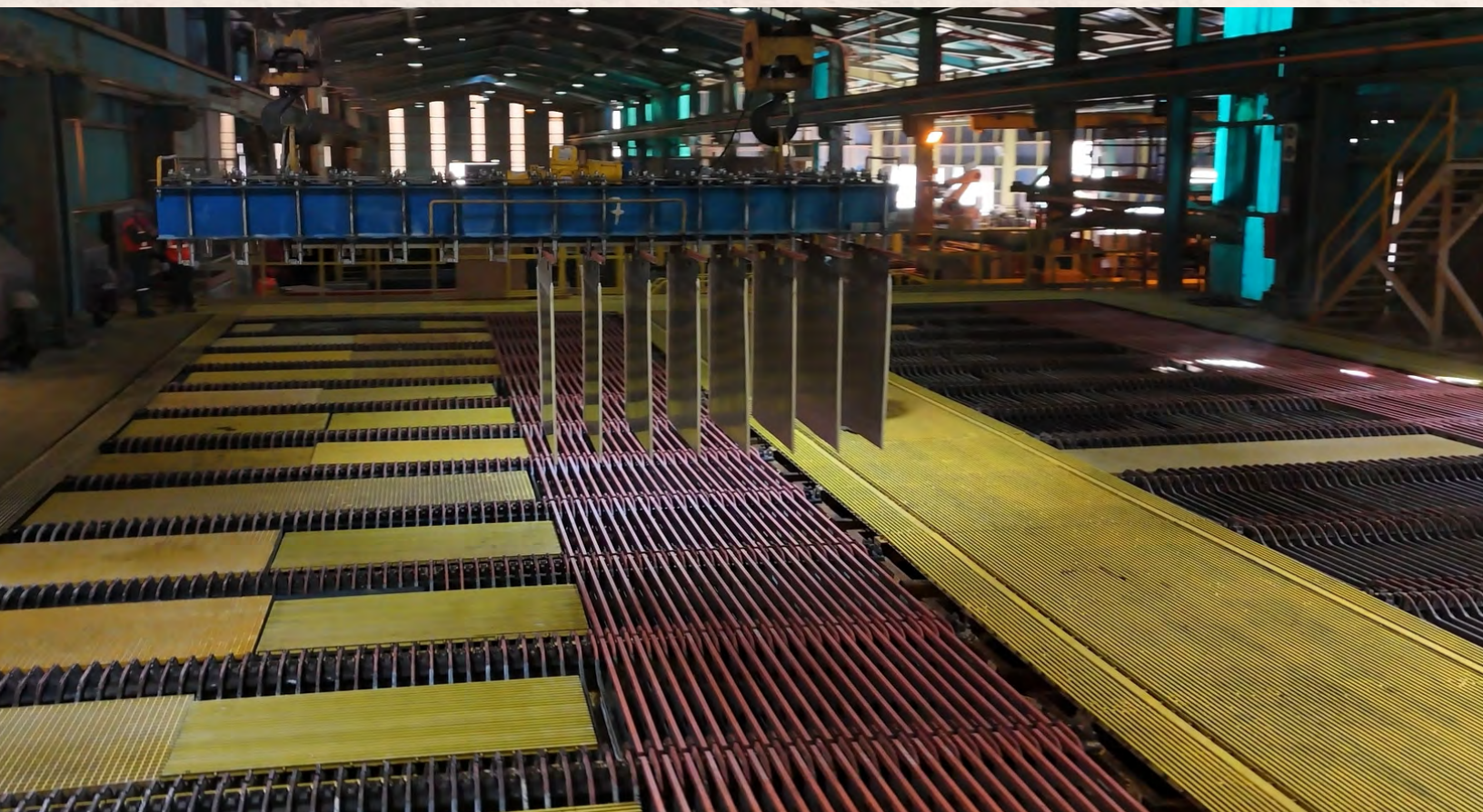
Mantos Blancos – Oxides Plant
