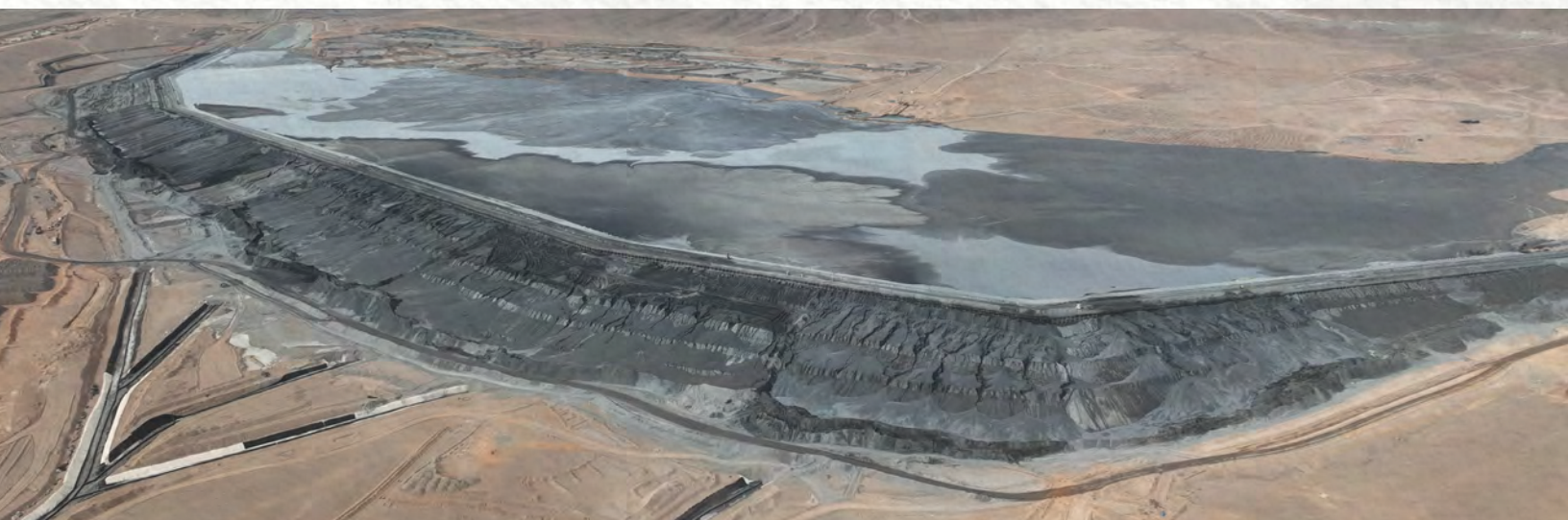
Mantoverde TSF – Construction of Sand Wall
