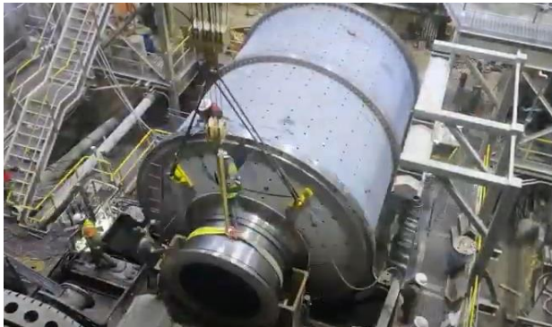
Pinto Valley Ball Mill Shell Replacement to Improve Reliability
