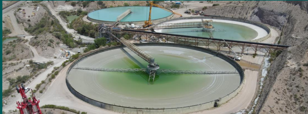
Tailings thickeners upgrades expected to result in increased water recovery and higher throughput.
