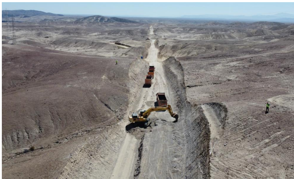
Early earthworks – By-pass of the C-17 highway
