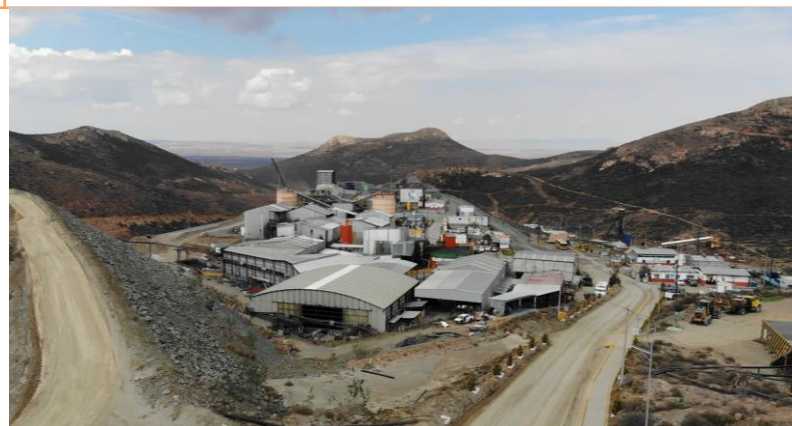
Cozamin – Commenced construction of paste backfill and filtered tailings plant
