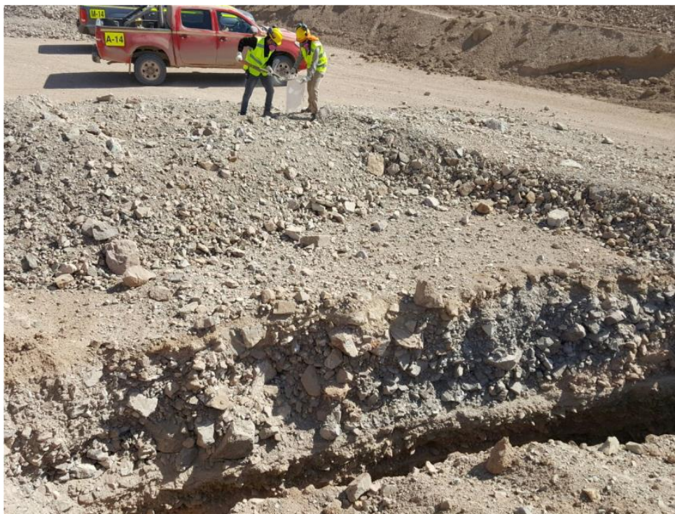
Figure 14-7: Trench Sampling of Mercedes Stockpile
