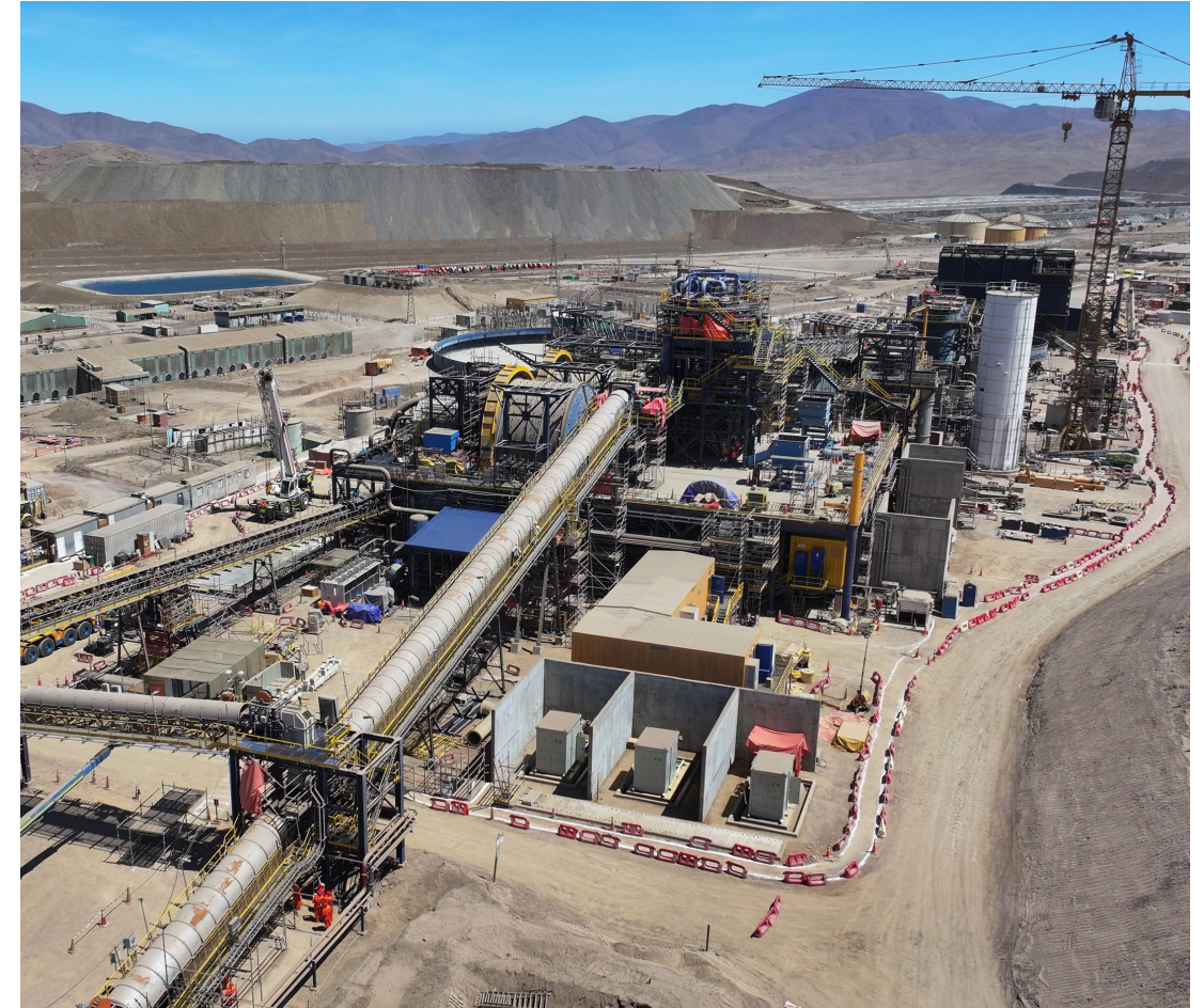
Mantoverde Development Project Processing View, October 2023.
