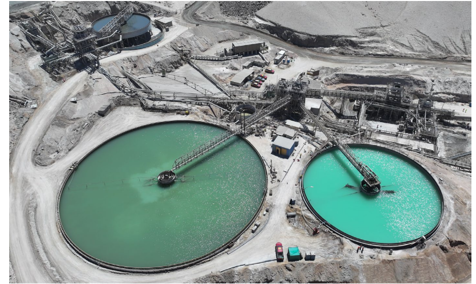
Pictured above is the tailings dewatering area of the Mantos Blancos mine. Debottlenecking of this area is a key focus to deliver a sustainable 20ktpd.
