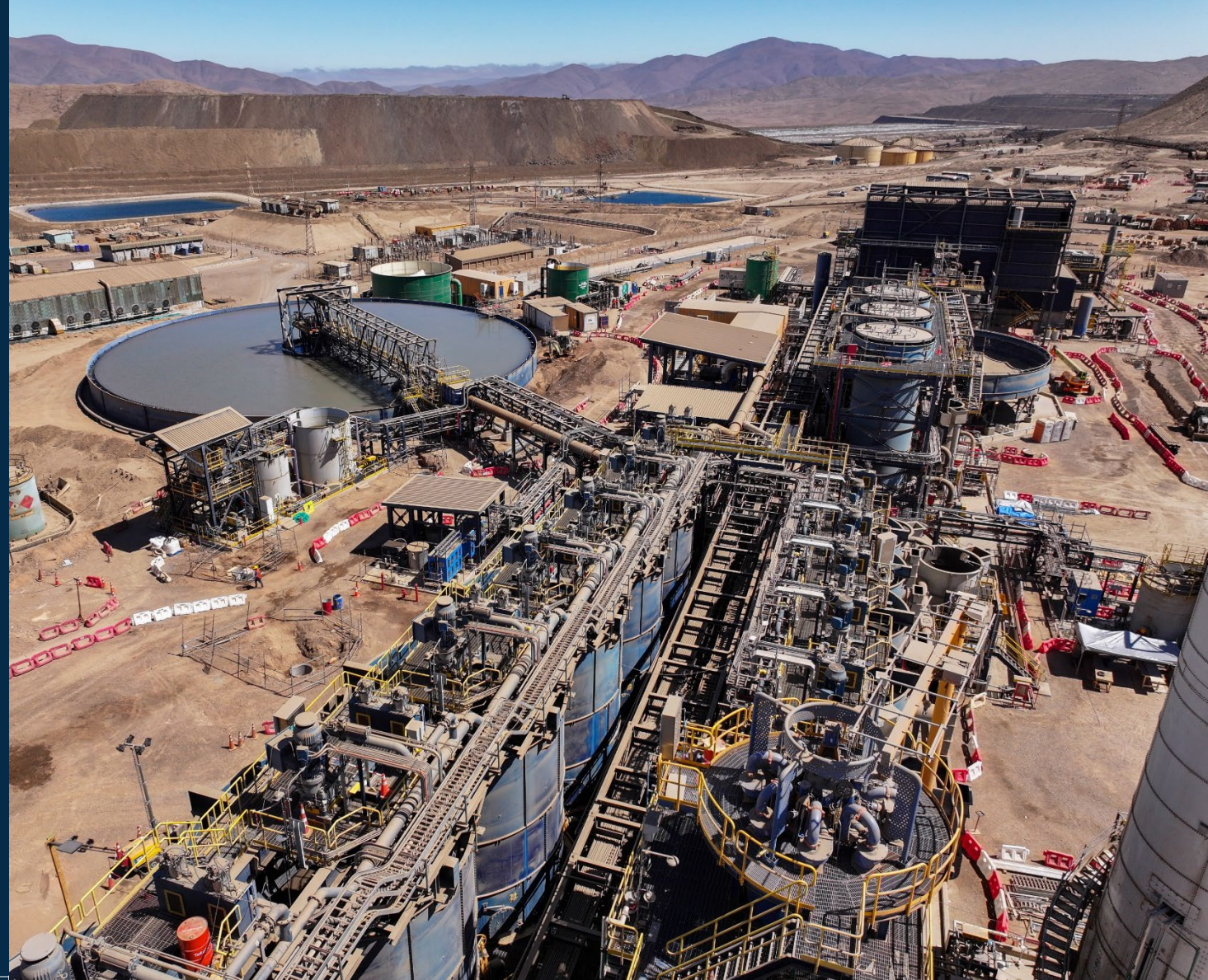
Mantoverde Development Project – March 2024
