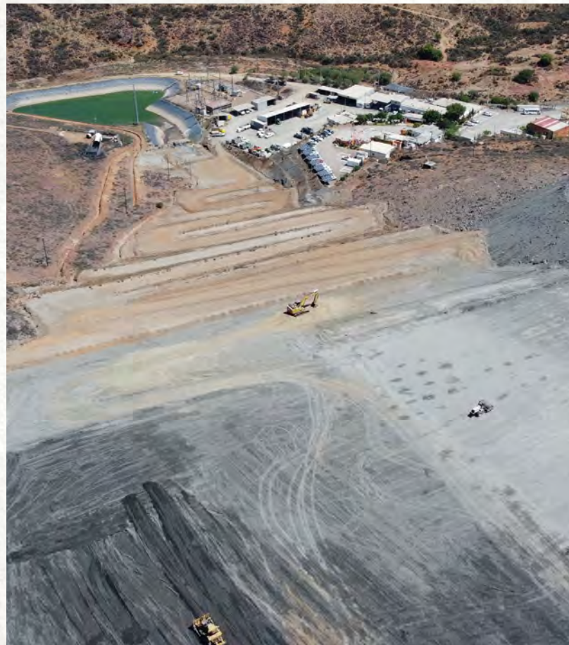
Cozamin – TSF Phase 1 with Partial Reclamation
