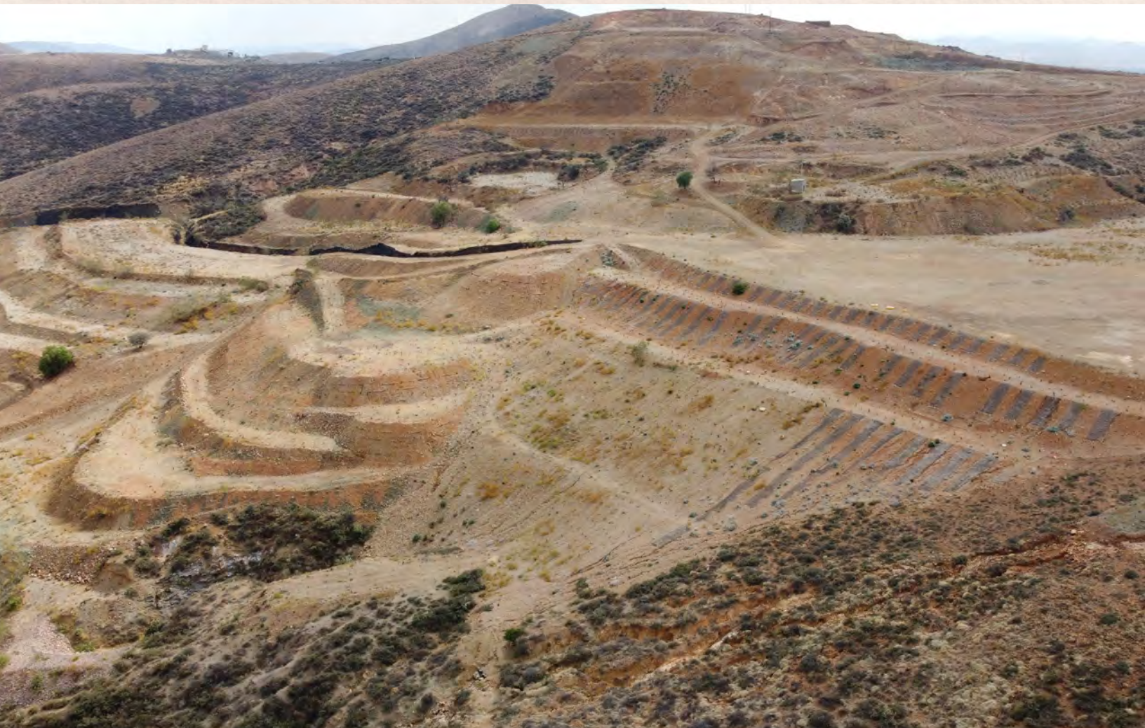
Cozamin – Chiripa TSF Reclamation
