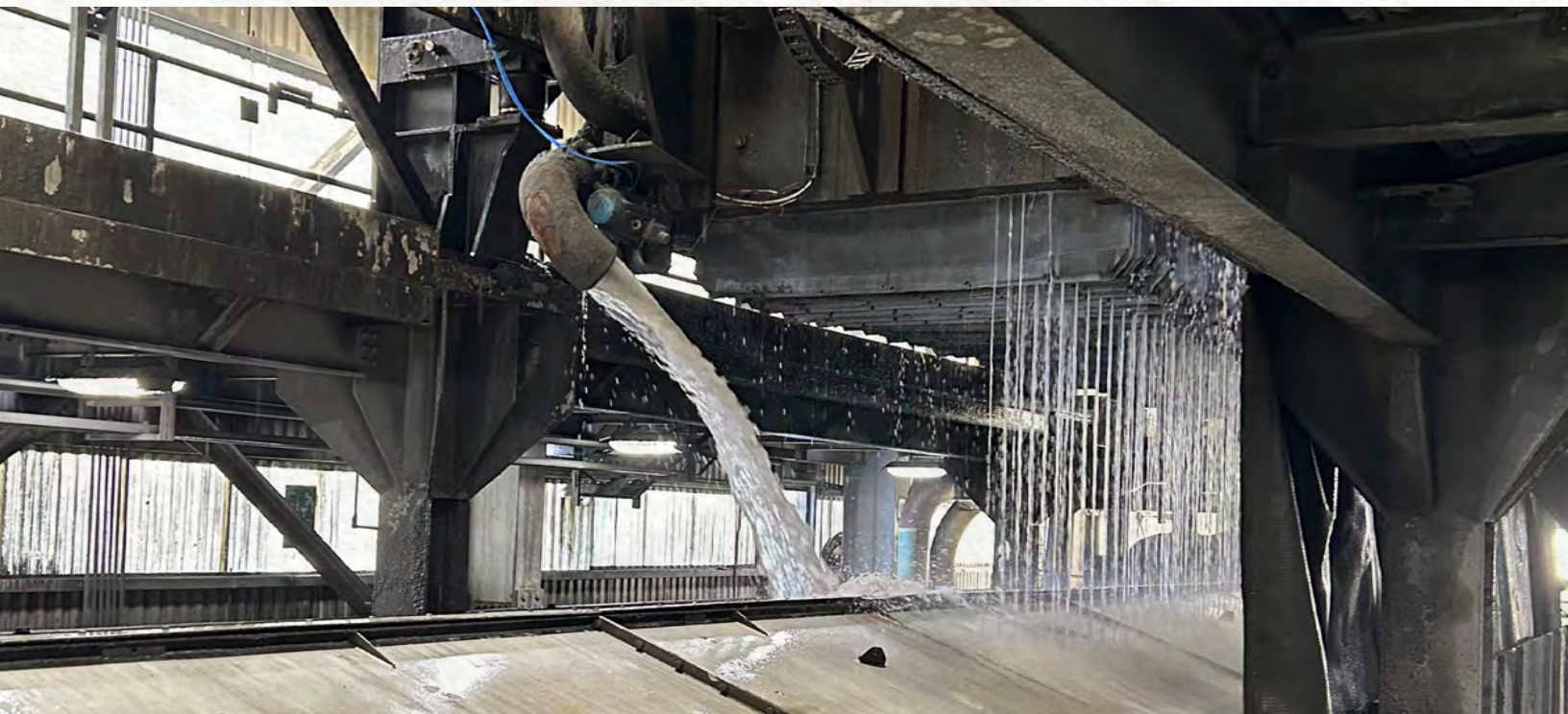
Cozamin - Water Recovery in Dry Stack Plant
