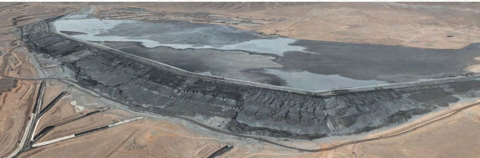
Mantoverde TSF – Construction of Sand Wall
