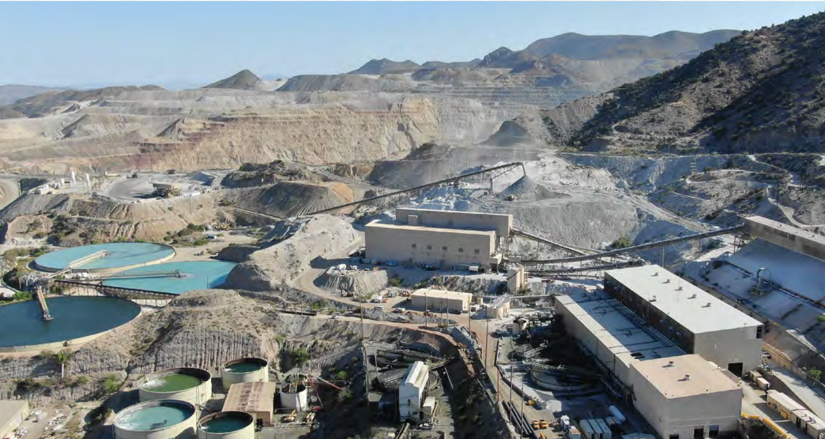
Pinto Valley – General View of Processing Plants
