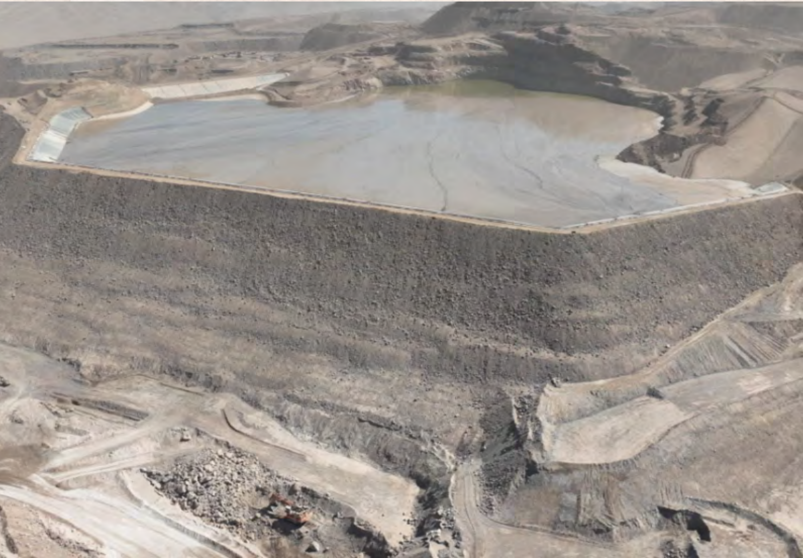
Mantos Blancos – Pit Phase 8, Stage 4 Construction
